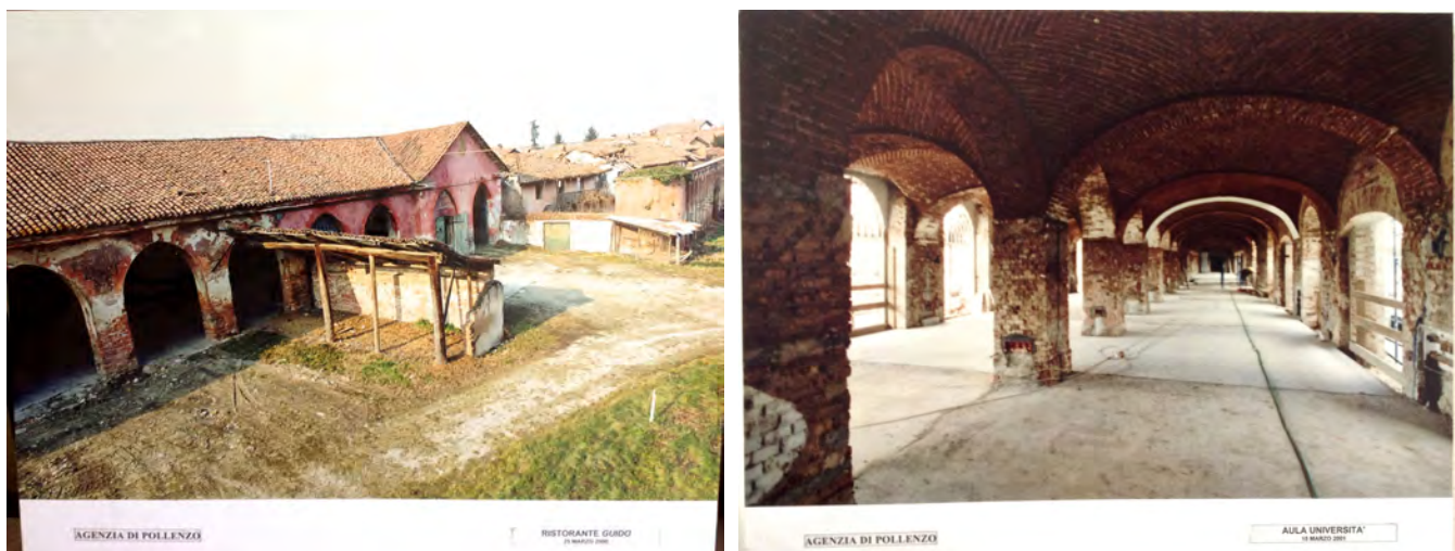
Fig. 5.2: posters depicting the state of the Agenzia di Pollenzo, prior to renovations in 2001; the stables (left) became the restaurant Guido, while storage areas (right) became UNISG classrooms
